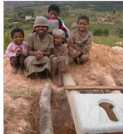
Members of a family of 15 who will share this improved latrine under construction. It includes a SanPlat, which HIP was instrumental in marketing and training masons to manufacture.
